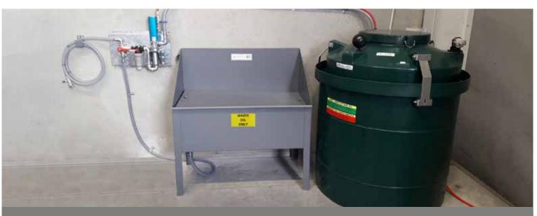
Waste oil Basin with pneumatic pump & suction filter. The pump kit removes waste oil from the basin and also mobile drain units, transferring in to the 1000L waste oil tank
