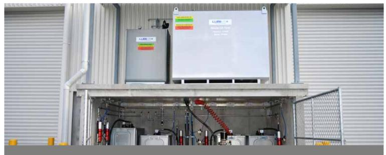
Bulk Oil Storage set up containing a 4500L Waste Oil Tank and 1000L Waste Coolant Tank
