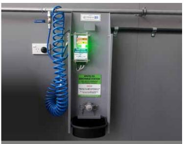
Waste oil drainer discharge station with incorporated drip tray
