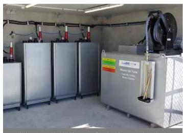
Lube store with 2000L waste oil tank with mounted suction hose reel and pneumatic waste oil pump. Typically suited for sucking from mobile service vehicles
