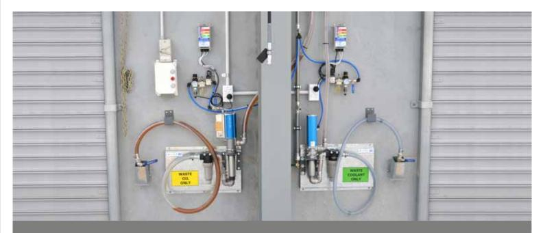
Waste oil & waste coolant drainer evac pump stations with pumps, suction filters and tank level alert systems
