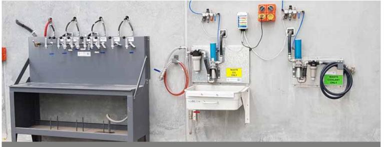
Wall-mounted Lube Pro 65L Waste Oil basin with Pump Station
