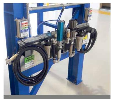
Waste Oil & Waste Coolant evac stations located at the end of a reel stand for easy access, with tank level alert system
