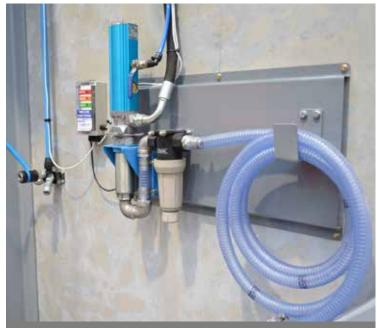
Waste Oil Pump Station with Tank Level Alert System
