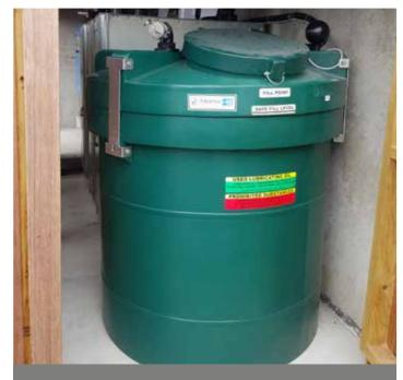
1000L Plastic Waste Oil tank with outer bunding tank, incorporated into tank room
