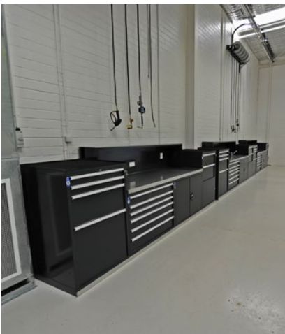
BAC Medium Profile Workstation, with various reels installed overhead
